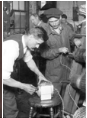
▲ Checking DC motor 1930
